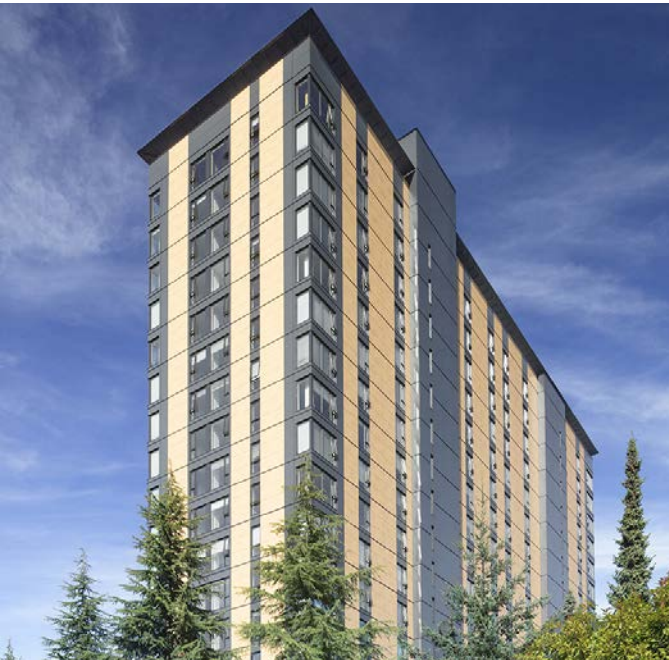
Photo: Michael Elkan, courtesy of Acton Ostry Architects
